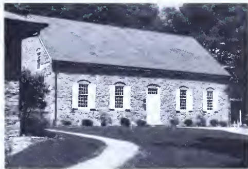
Paxton Presbyterian Church (c. 1740), Paxtang Borough, Dauphin County; limestone and dolomite (St. Paul Group) from local quarry.
